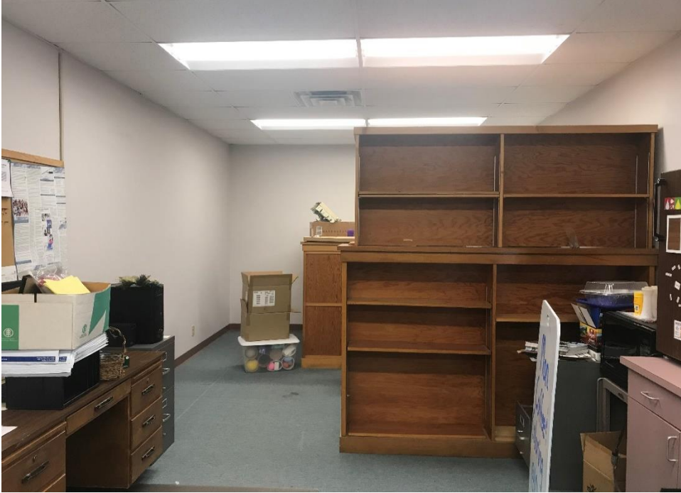
Figure 1: Before Backroom Remodel
